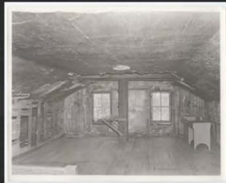
Attic of the East Building, circa 1939. The SIMLS used the attics of the East and West buildings as student dormitories. Photo courtesy of the Kansas State Historical Society.
